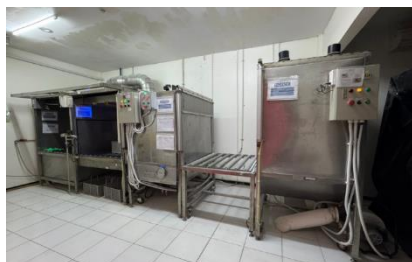
Gambar 4. Penetrant Line System
