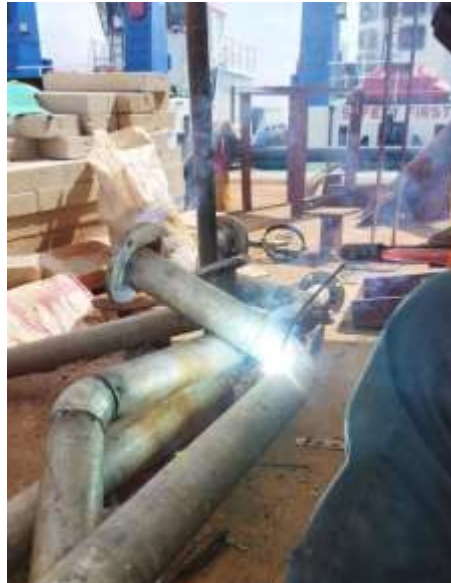
Gambar 5: Proses fit-up dan alignment pipa
