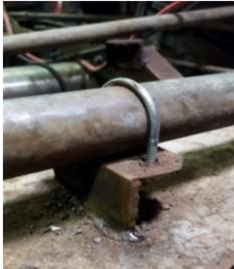
Gambar 7: Proses pemasangan pipe support
