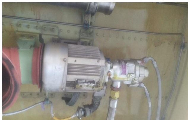
Gambar 8. Standby Hydraulic Pump
