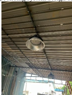
Figure 11. Lighting and High Bay Installation, Workshop 3 & 4, PT VME Process
