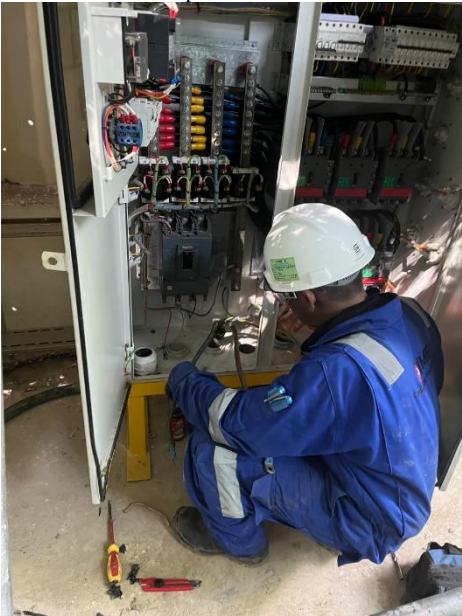
Figure 8. Panel Installation and Termination (LV.MDP / SDB / DB), Workshop 3 & 4, PT VME Process
