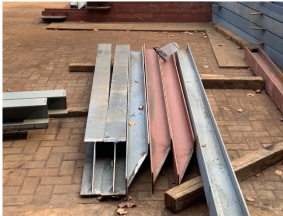
Gambar 6: Hasil Potongan H beam
