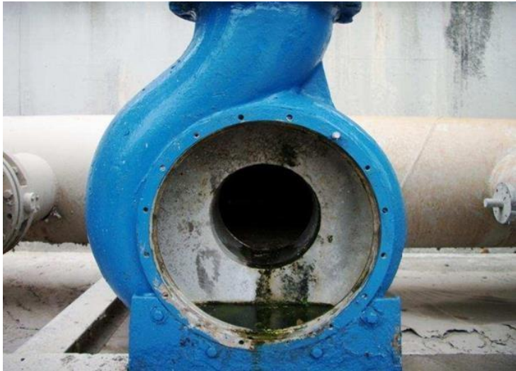
Gambar 2. 3 Casing Pompa Centrifugal
