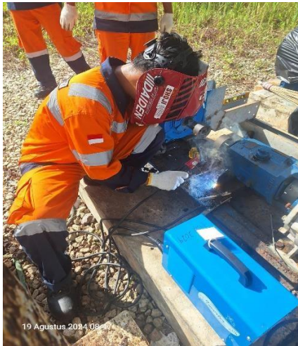
Lampiran 4 pengelasan support pompa demin B
