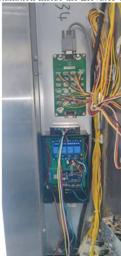
Figure 17. Hardware Installation Inside the Elevator Control Panel
