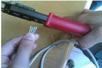
Gambar 2.5 Proses Cutting
