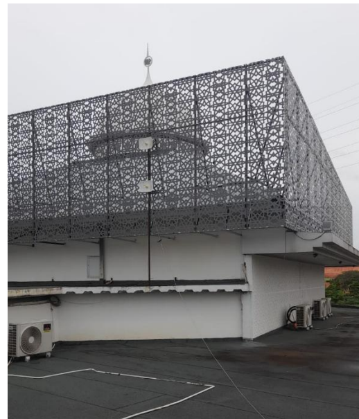
Figure 3. Roof Lighting Near the Mosque Dome
