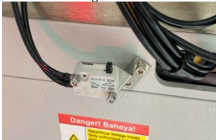
Figure 11. Implementation of Semi-Automated Cleaning System
