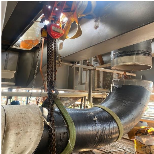
Gambar 3. Preparasi Pipe Spool
