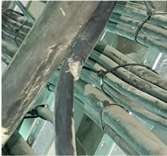
Figure 9. Cable Damage
