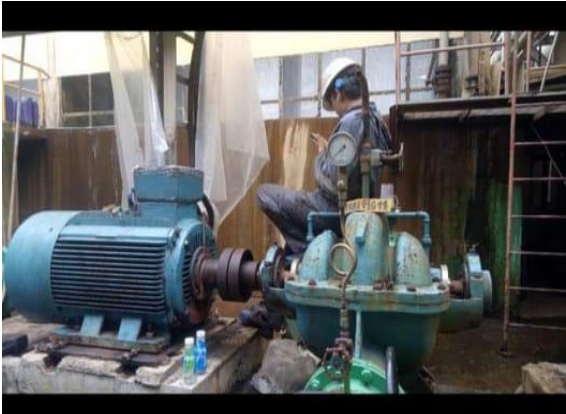
Lampiran 5. Repair icw pump A
