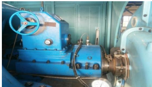
Gambar 2.9 Turning Device
