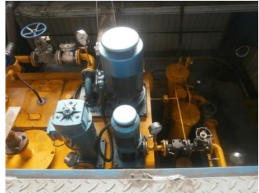
Gambar 2.11 Oil tank, Oil filter dan Oil pump
