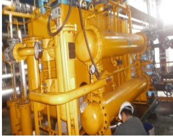
Gambar 2.11 Oil tank, Oil filter dan Oil pump
