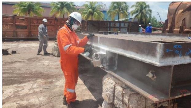
Gambar 5: MPI lifting lug sesudah Load Test
