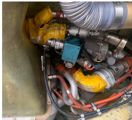
Gambar 10: Pack valve installed
