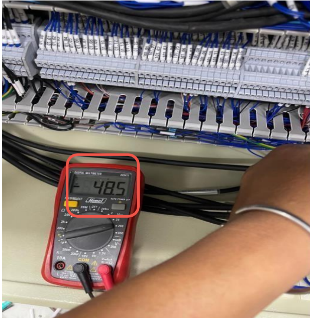
Gambar 38 Pengecekan Sumber Tegangan 48VDC
