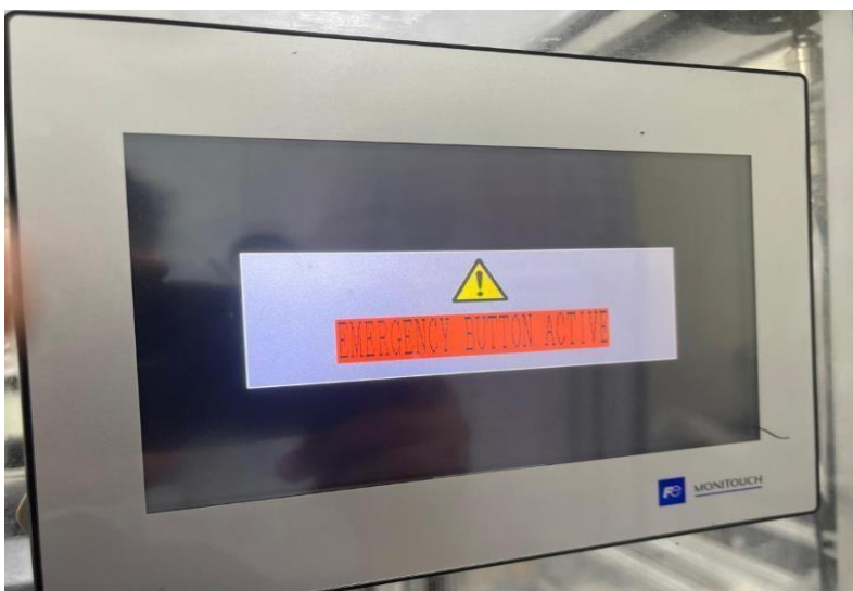
Gambar 60 Display HMI Emergency
