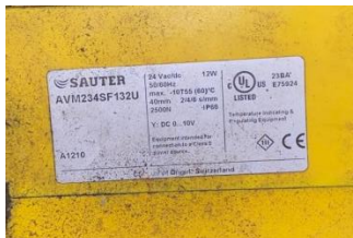
Gambar 8. Nameplate Motor Servo SAUTER
