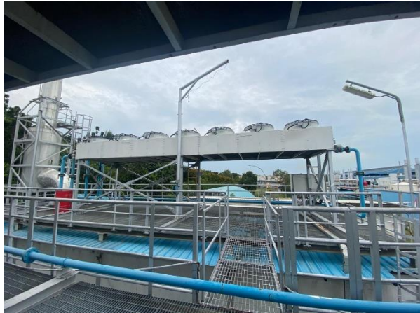
Gambar 11. Radiator PLTMG Batamindo
