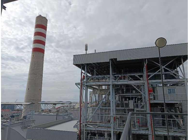
Gambar 1 PLTU PT. Bintang Alumina Indonesia (BAI)
