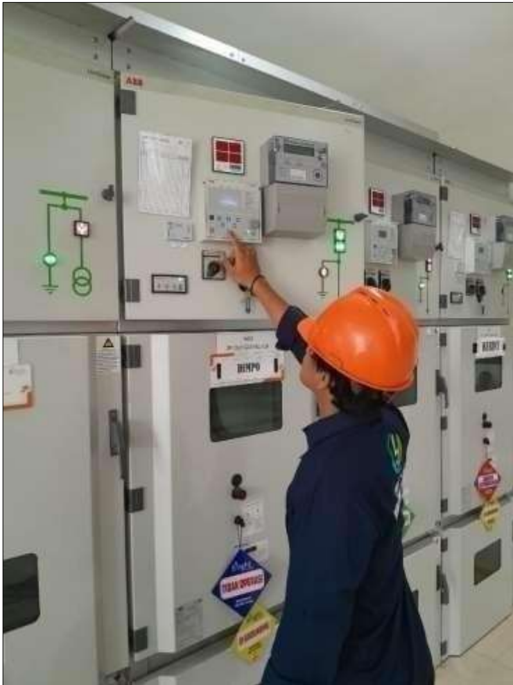
Gambar 1. Gangguan indikasi trip circuit
