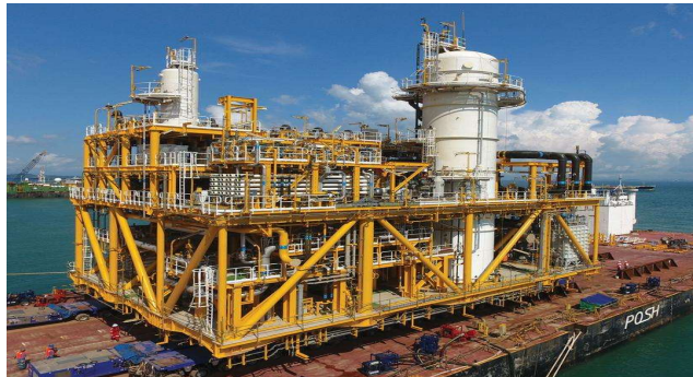
Gambar 1.2 Modules, skids, and platforms
