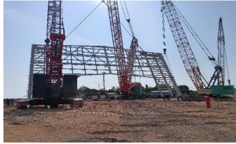
Gambar 3.7 : Proses Tailing Lifting
