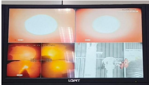
Gambar 11. Fouling Sesudah di Sootblower di Distributed Control System
