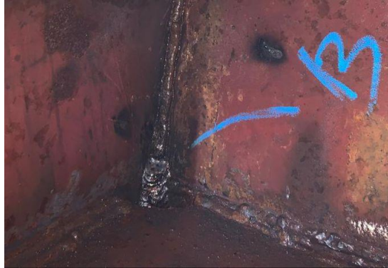
Gambar 5. Contoh penambalan kebocoran
