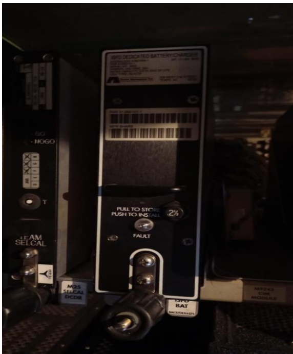
Gambar 17. ISFD Dedicated Battery Charger
