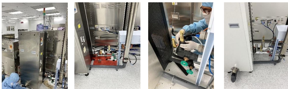
Gambar 9 : Fabrikasi chilled water & exhaust
