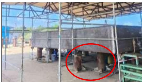
Gambar 2. Struktur Stool (Temporary Structure)
