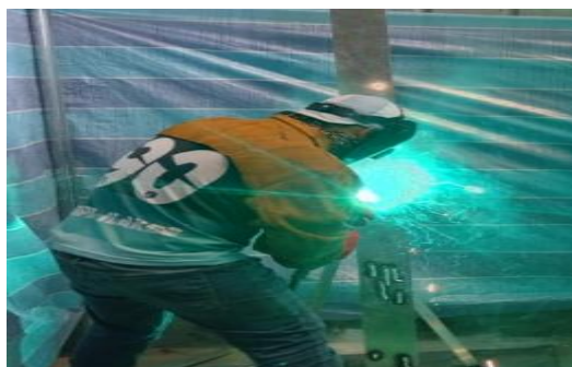
Gambar 11: Pengelasan 3G
