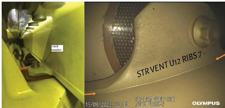
Gambar 7: Crack Upper Vent Stringer 12A Rib 7
